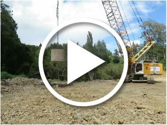
Both these methods increase the strength of the soils and prevent them liquefying during earthquakes. Liquefaction damages bridge foundations.
