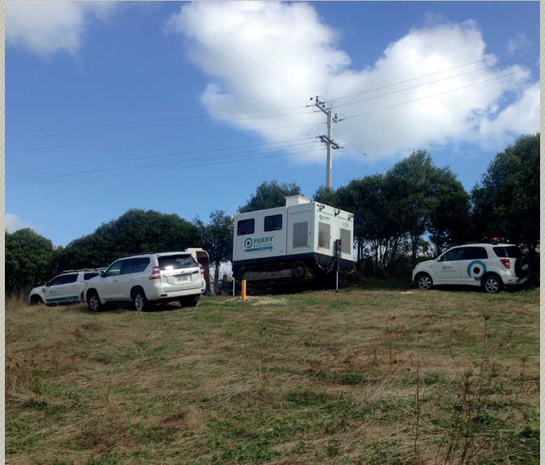
Geotechnical investigations are under way across the project
