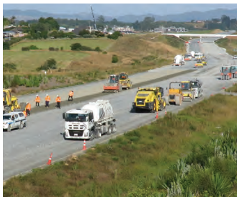
Cement stabilising in progress near Gordonton Road.
