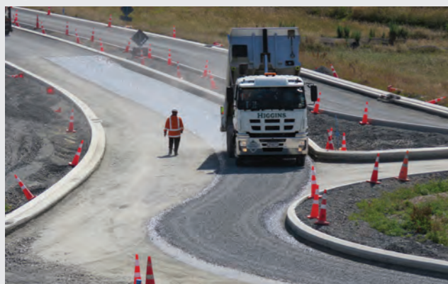
The roundabouts at the interchange were chip sealed in January, which completes the chip sealing along Pardo Boulevard. A final layer of thick asphalt is still to be laid over the chip seal. South of Greenhill Road, a second stretch of Hi-Lab road rock is being laid and stabilised.
