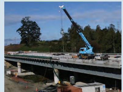
Barriers are being installed on the Mangaonua Stream Bridge.
