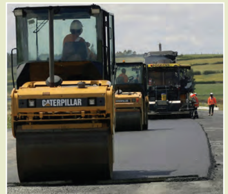
Rollers compact the asphalt and smooth the joints.
