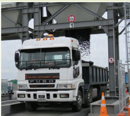
Trucks drive under a hopper at the asphalt plant and are filled automatically.
