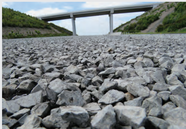
The four lanes under the bridge are now chip sealed and ready for asphalt.
