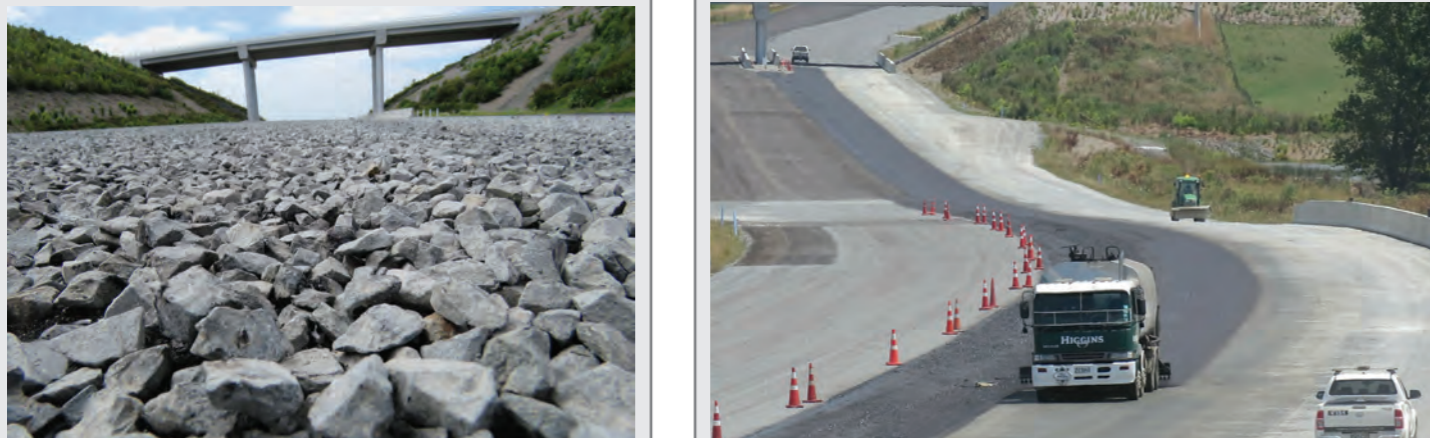
The four lanes under the bridge are now chip sealed and ready for asphalt.
