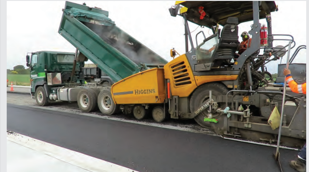
The final asphalt is being laid at the Ruakura Interchange to enable the Ruakura West road connections to be constructed. Trucks building the roads that will connect the interchange with Silverdale Road and Ruakura Road will use the interchange for access.
