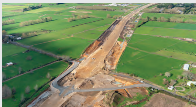
Construction of the ramps to take the expressway over the Powells Road underpass is now complete. The weight of the embankments will now cause the soils beneath to settle. Once settlement targets have been achieved, the site for underpass will be excavated, the ground strengthened and the concrete structure constructed.
