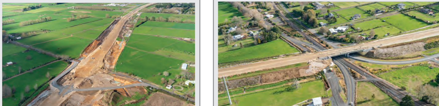
Construction of the ramps to take the expressway over the Powells Road underpass is now complete. The weight of the embankments will now cause the soils beneath to settle. Once settlement targets have been achieved, the site for underpass will be excavated, the ground strengthened and the concrete structure constructed.
