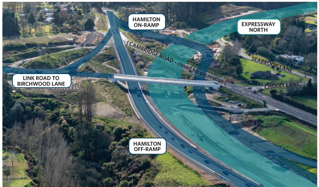
The photo in this illustration shows traffic flowing on the new lanes under the East West Link Bridge. These lanes will eventually become the two-lane off-ramp to the city. The illustration also shows the final location of the four-lane expressway and the on-ramp heading south from the city.
