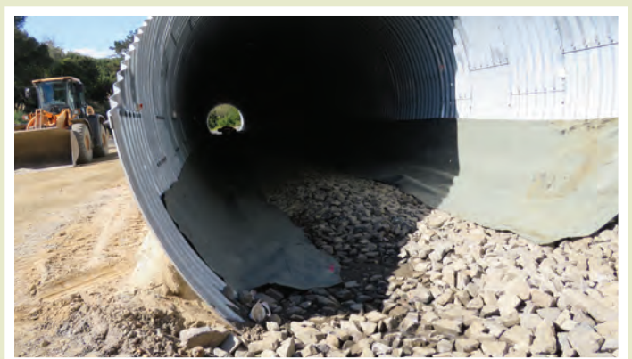
Construction of a stream bed inside the culvert has begun.
