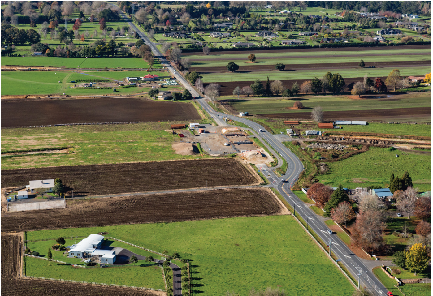
An aerial view of Matangi Road Bridge construction looking west to east along Matangi Road taken early June 2017.
