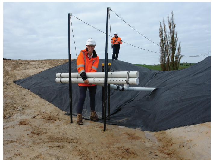
Checking a decanting pond outlet.
