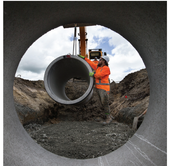
Before we install culverts, we capture and relocate native fish
