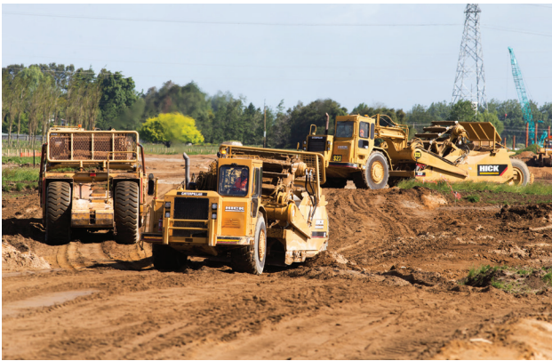
Earthmoving machines move sand to form the Ruakura Interchange
