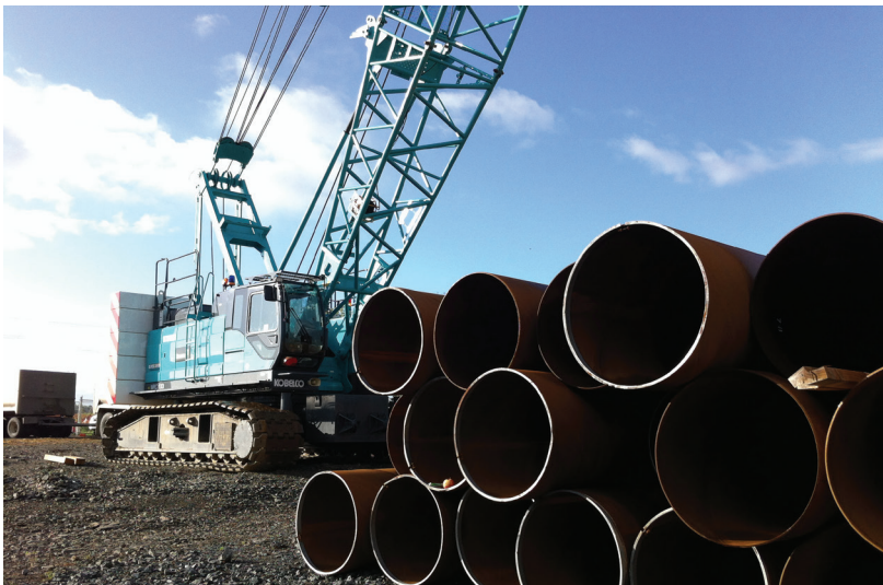
Our 100 tonne piling crane
