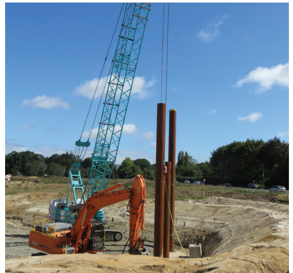
Piling in progress
