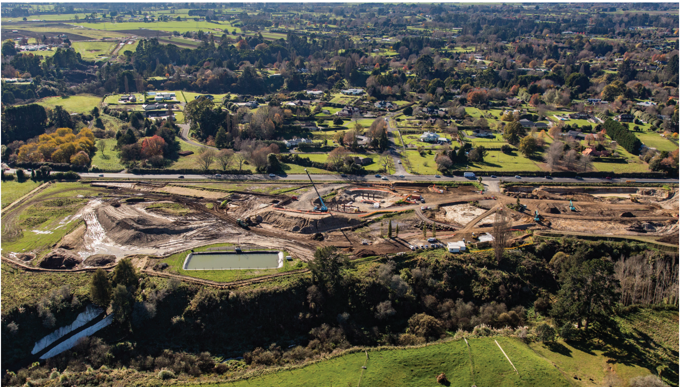
East/West Link Bridge taken early June 2017
