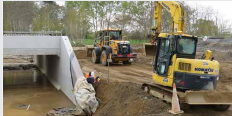
Fill is being placed either side of the Resolution Underpass.
