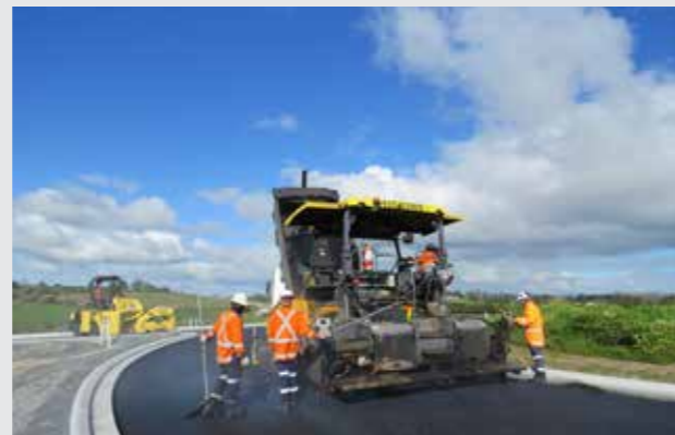
Laying asphalt at Resolution Interchange.
