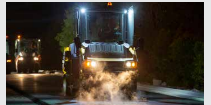
Asphalt being laid at night.
