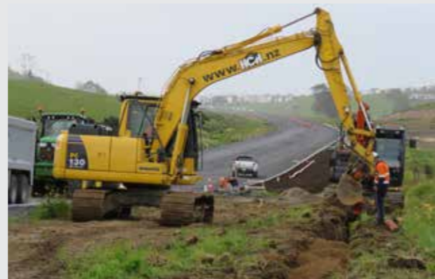
Drainage being installed on the extension to Resolution Drive.
