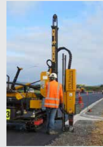
Sleeves driven into the road will support flexible (wire rope) barriers.
