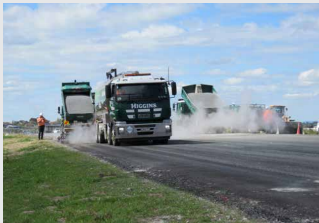
The bridge is complete. Landscaping continues. Prime coat spraying and chip sealing is under way. Work is about to resume on the link from the interchange to Resolution Drive.
