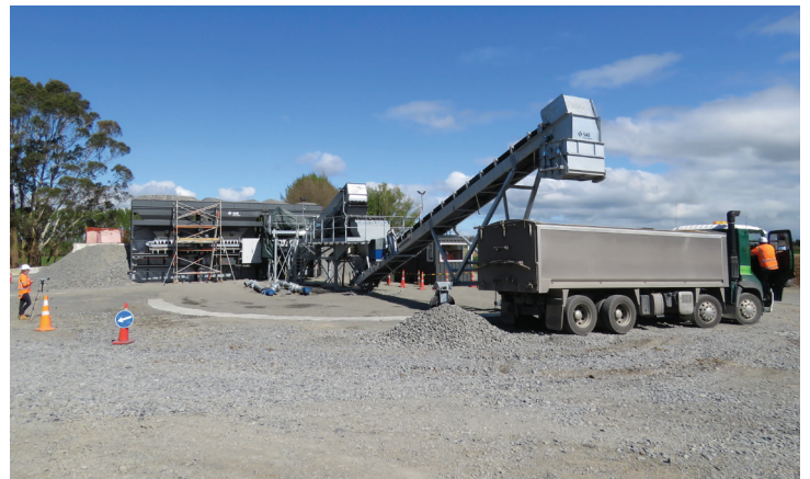
The blending plant in action at Lake Road.
