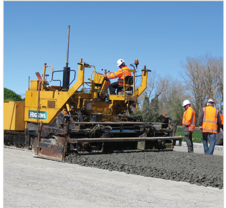
Hi-Lab pavement is tested at the Southern Interchange.
